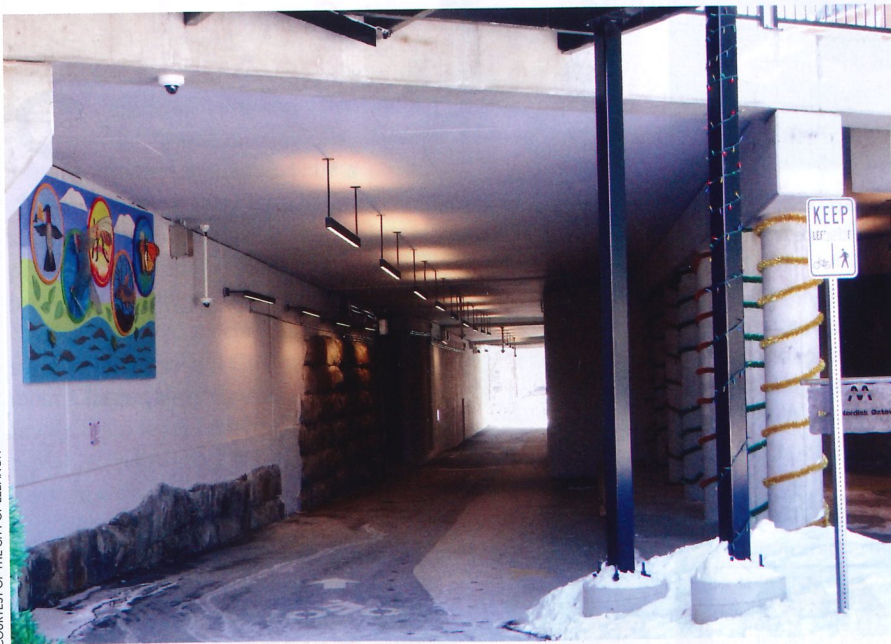
The rail trail tunnel features public art installations.
